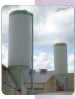
Silo diameter 2.4m Dome height 0.6m Cone depth 1.95m Cone angle 60°
